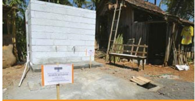
A water storage unit and infiltration well in Dusun Jatian
