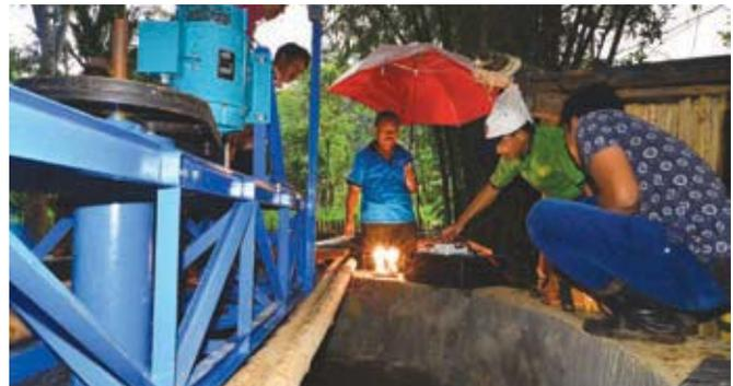
*Installing the turbine and other equipment at a micro hydro site in a rural area near the Paiton II Power Station, Indonesia*
