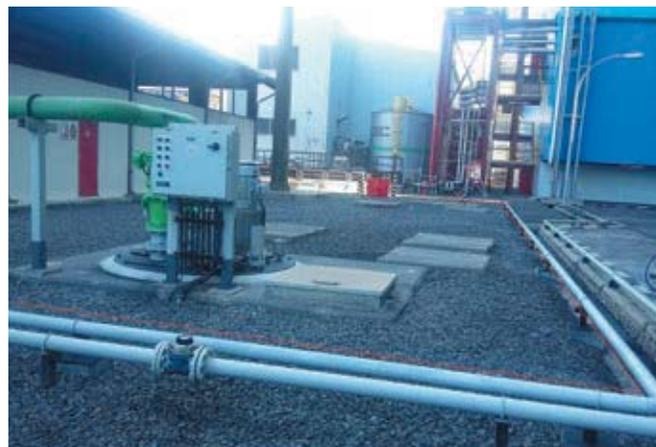
*New pipeline installed at Paiton II Power Plant, Indonesia to direct recycled water from the sampling panel feed water to the reverse osmosis unit*
