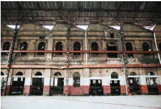
⤴ The historical Sentul Depot located at the heart of Sentul West was Kuala Lumpur’s best kept secret until it was unveiled again in its 113-year history. The depot with its stunning colonial-brickwork is rich in heritage and history dating back to 1905. It used to be the largest complex of railway workshops which once served the Federated Malay States Railways in the early 1900s up to the KTM era in the early 2000s
