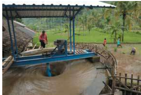
⚡ One of the micro hydro unit installations at Sumberejo Village at Situbondo regency, Java by YTLJT team
