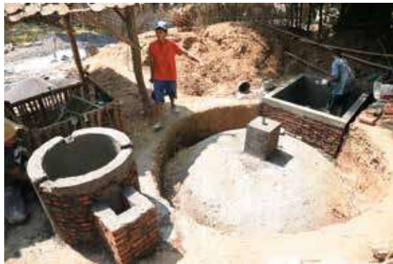
⚡ A dome-shaped reactor functions as a digester where biogas is generated from the decomposition of cow manure. The residual sludge from the digestion process will be used as fertiliser for agricultural purposes
