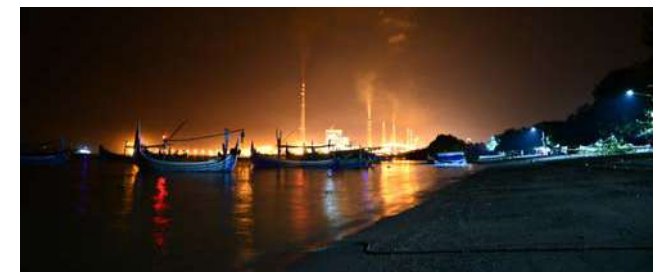
Solar cell lamps installed at Bhinor Fishing Harbour provides lighting for the fishing community
