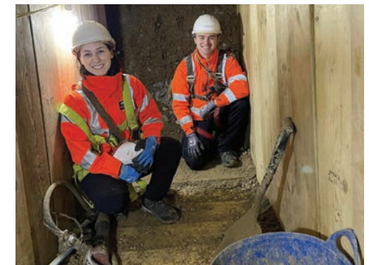
Fran Thums and a colleague heading tunnel repairs during on-site work
