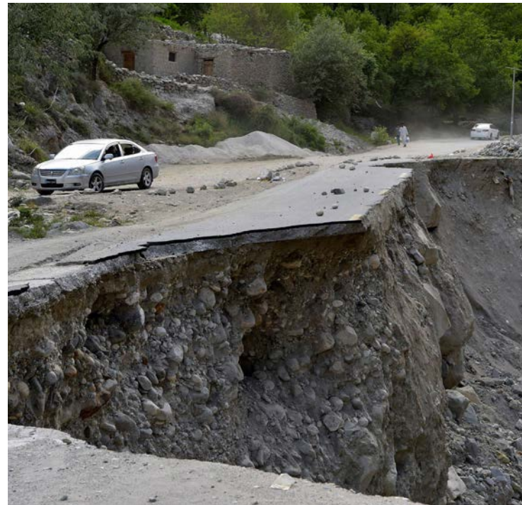
A high flood from the Shishper Glacier severely damages a section of the Karakorum Highway in Pakistan, September 2022 (photo by CNN)
