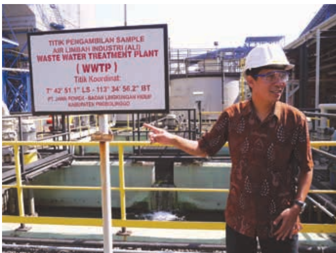
Effluent is processed and recycled at YTLJT's wastewater treatment plant
