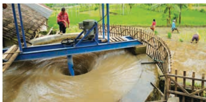
— A micro hydro unit at Sumberargo village, Situbondo regency, handed over in February 2018
