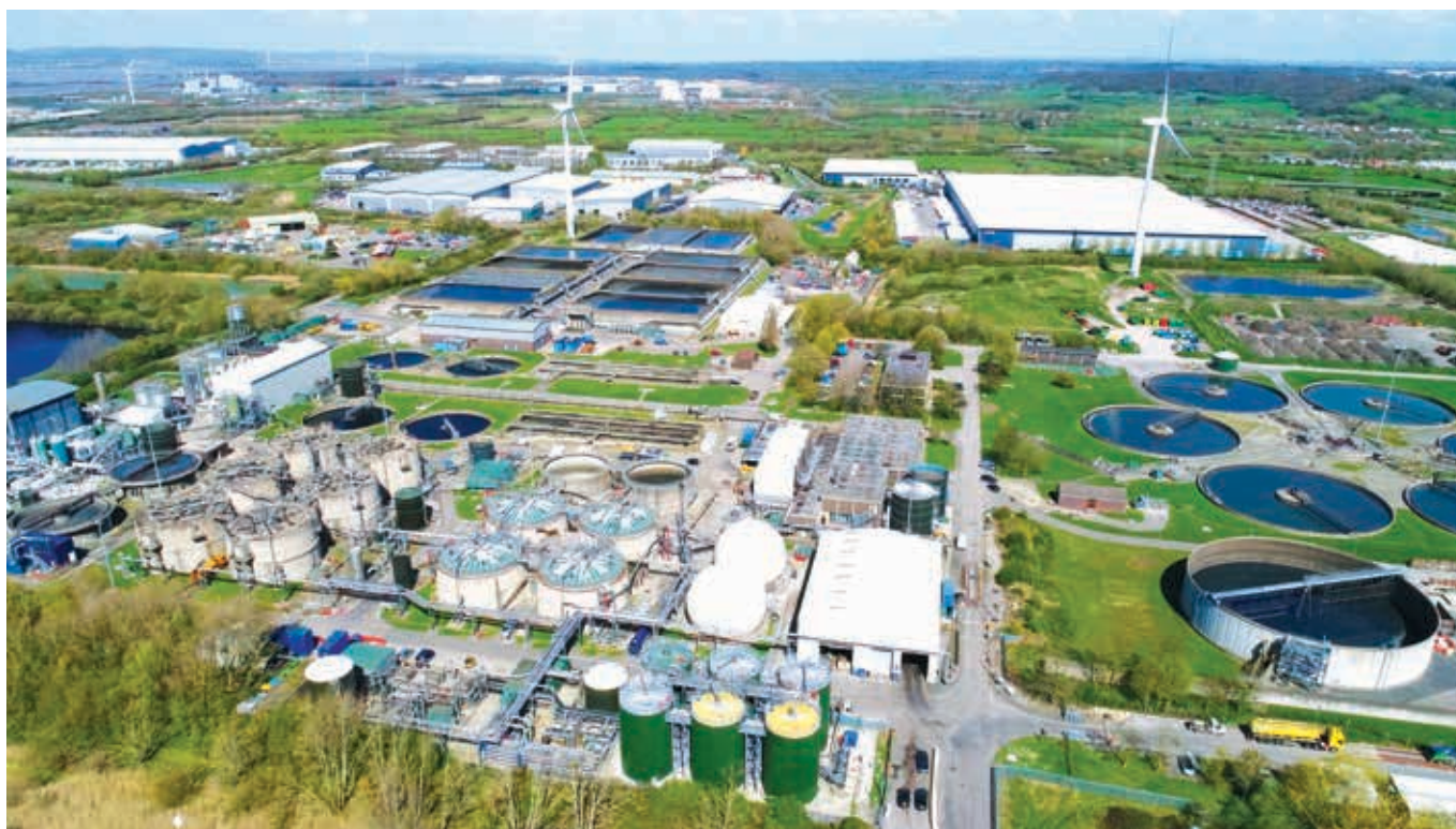
— The wastewater treatment plant in Avonmouth, which is operated by GENeco, treats 75,000,000 m 3 of sewage waste every year
