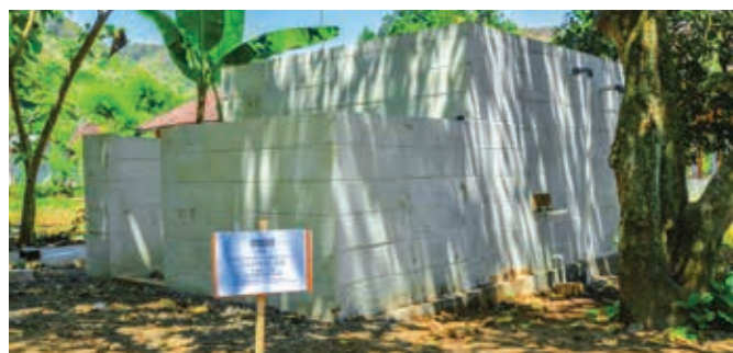
One of YTLJT's water conservation programmes where an additional water storage unit was installed and utilised by 30 families from Selobanteng Village
