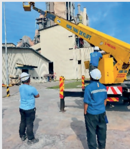
Skylift Inspection to ensure all safety devices are functional before use
