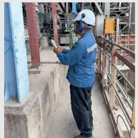
Noise level monitoring to identify high noise areas in the plant
