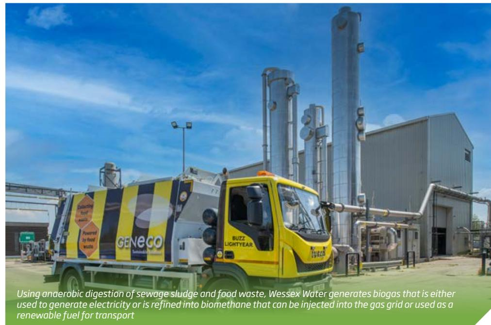
Using anaerobic digestion of sewage sludge and food waste, Wessex Water generates biogas that is either used to generate electricity or is refined into biomethane that can be injected into the gas grid or used as a renewable fuel for transport
