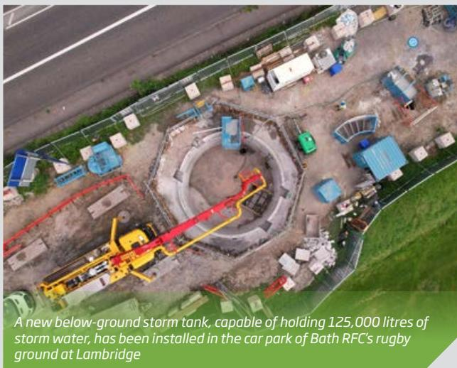
A new below-ground storm tank, capable of holding 125,000 litres of storm water, has been installed in the car park of Bath RFC's rugby ground at Lambridge
