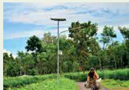
Street lighting was replaced with solar cells at the OHC entrance
