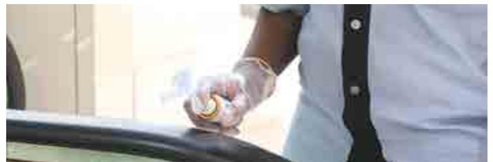
Antivirus, antimicrobial and antifungal coating applied onto escalator handrails and lift buttons
